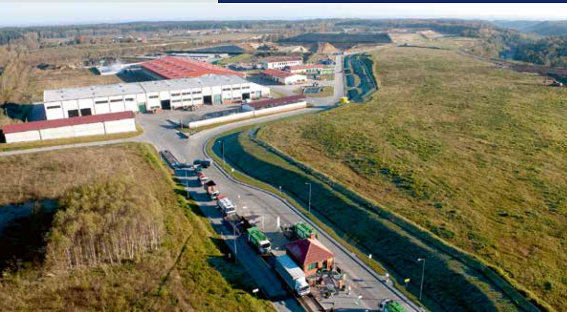
EcoValey - Gdynia recycling and waste utilisation plant
