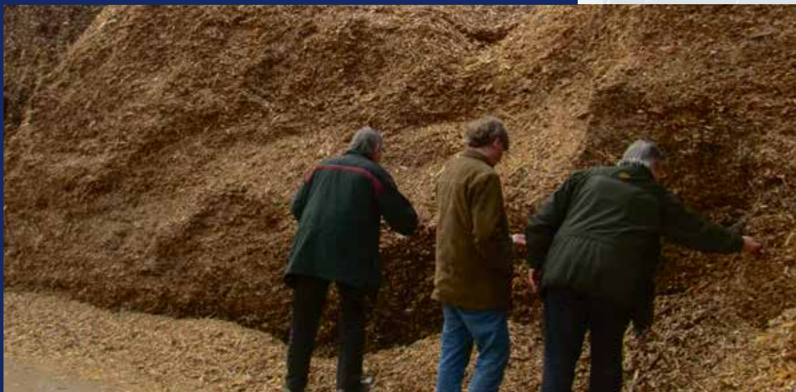
Wood chip storage at the district heating plant in the city of Ludza
